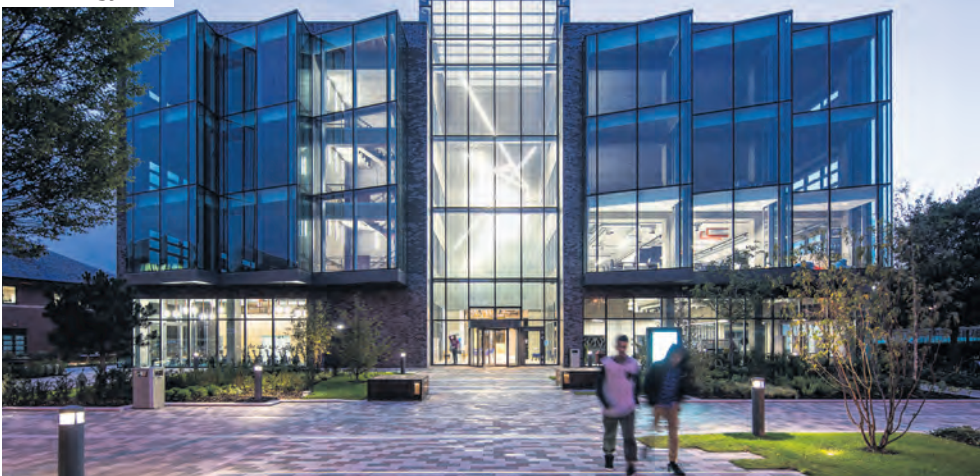
Bright Building, a 'living lab' for state-of-the-art technology
